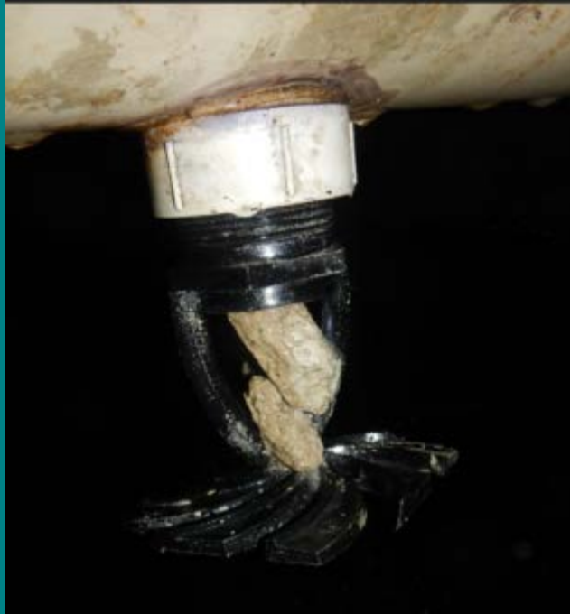
Water distribution nozzle spray clogged by sulfur and silica deposit
