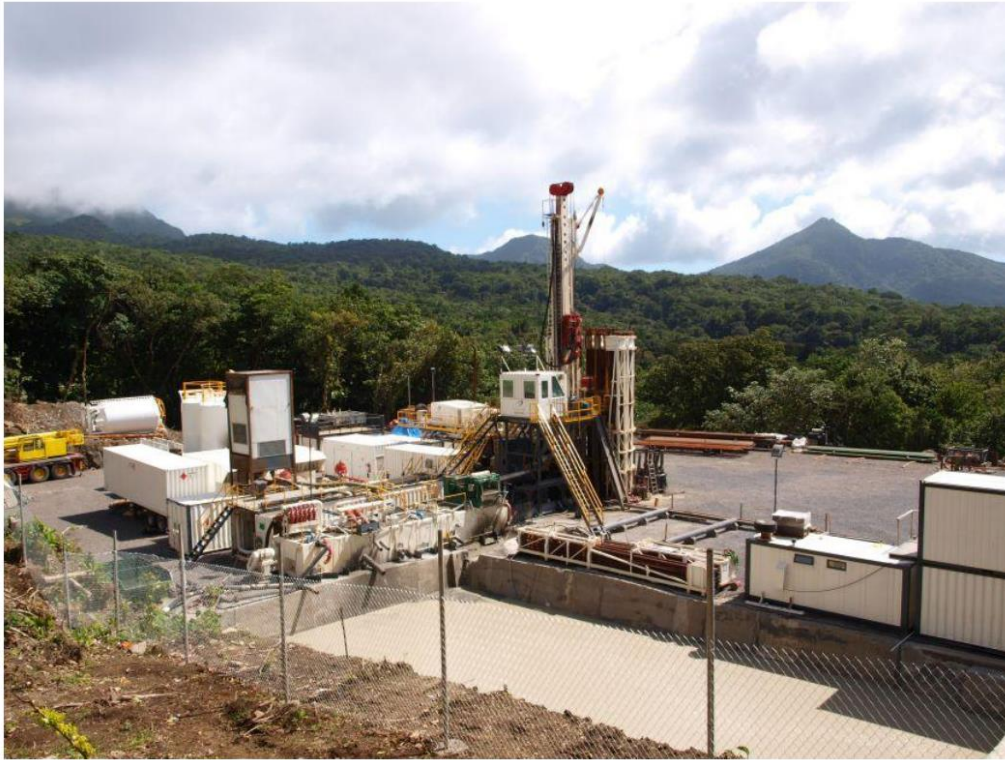
Figure 5 Rotary rig (100 t) drilling slim hole to 1500 m (Source: ISOR)
